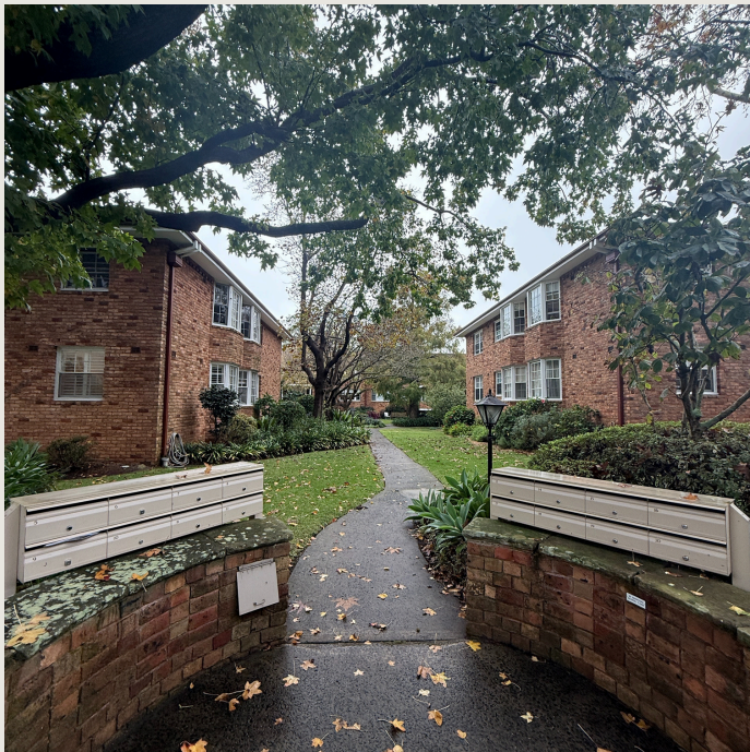
4 Neighbouring Buildings at 2 Cherry St.
