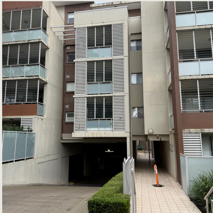
5 Neighbouring Buildings at 3-13 Cherry St.
